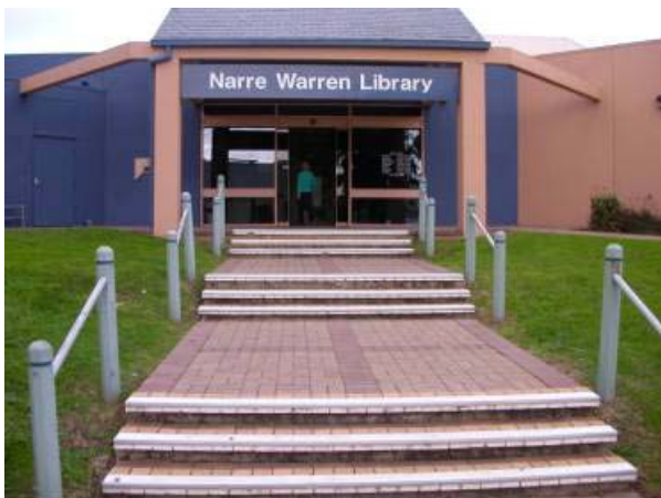
Photograph 24 High CCAT Entrance
