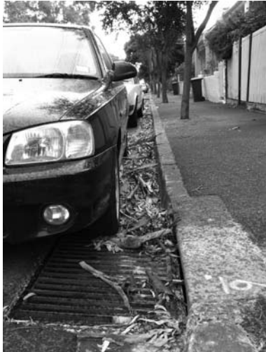
Leaf and tree litter at risk of being washed into the stormwater drain.
