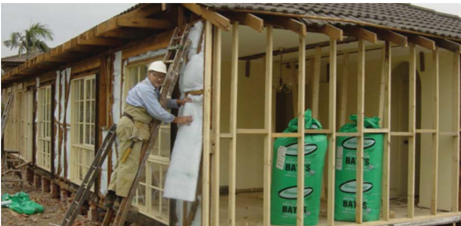
Carmine Bernardo of Better House Removers says his company is already making the homes they relocate more sustainable. One way is insulating brick veneer homes, like the one pictured.
