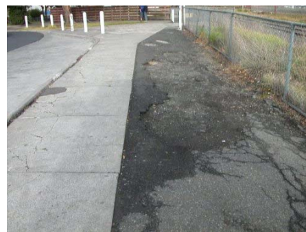
Photo 9 Open space surfaces not level
